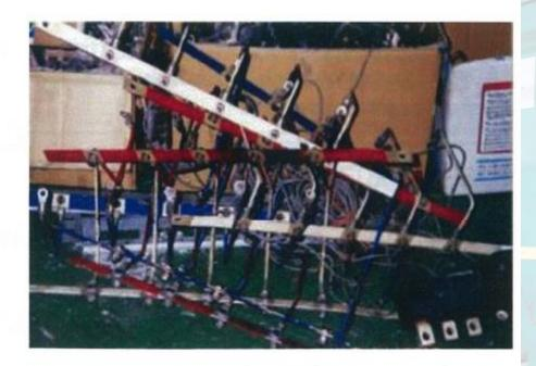
Most of electrical parts in 440V feeder panel became nonusable
