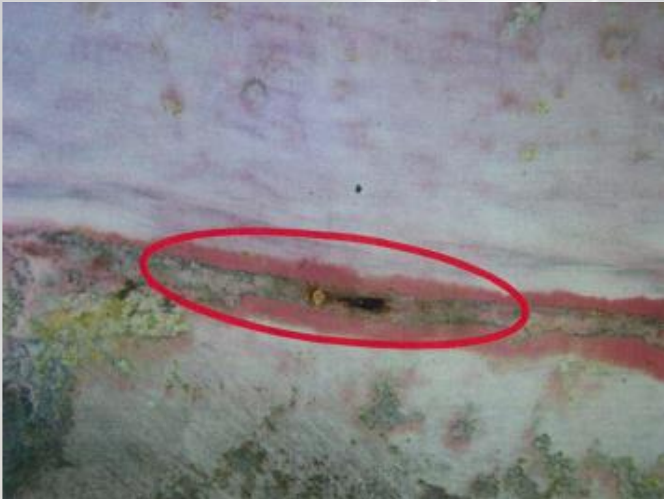
Leakage from Double Bottom Tank
