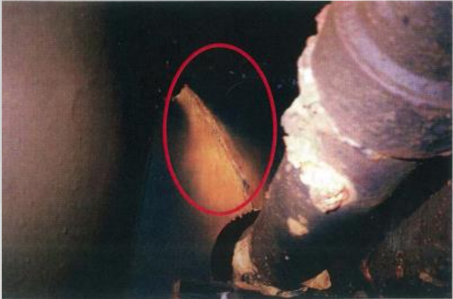
Crack in pipe penetration
