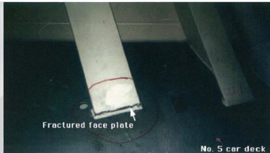
Fractured side Frame
