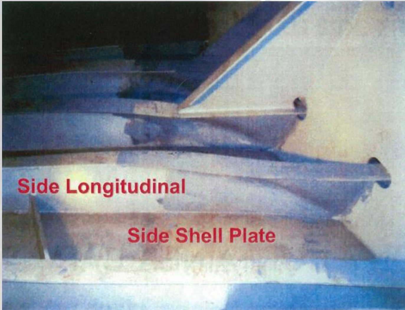
Buckling at Side Longitudinal & Side Shell Plate
